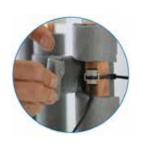
Each TMU accepts up to 4 temperature probes (configured as 2 pairs) which simply affix to pipe work surfaces using clips (15mm) or cable-ties (>15mm).
